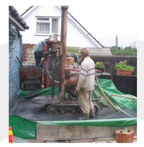
A borehole basically consists of a hole drilled between 60 and 100m deep vertically down. Generally the borehole diameter is around 110 - 145mm, but this diameter depends on the type of machine being used to drill the borehole and the diameter of the borehole pipe (usually 32-40mm). The drilling rigs used by drillers come in many shapes and sizes some small enough to operate and gain access to small gardens others designed for larger commercial projects.
