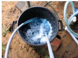
Fig 15 Purging the arrays of air
