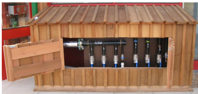
Fig 7 Header manifold connections
