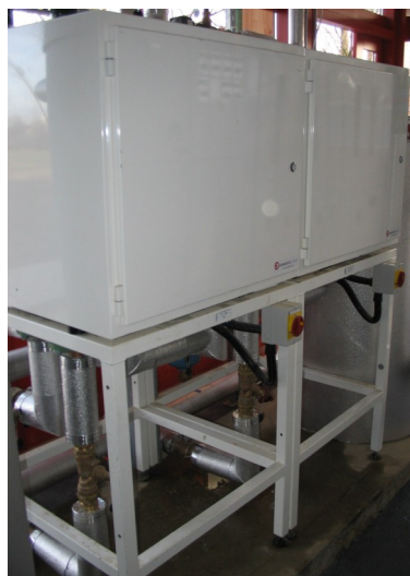
Fig 6 Plant room heat pumps
