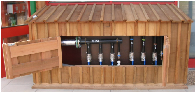
Fig 7 Header manifold connections
