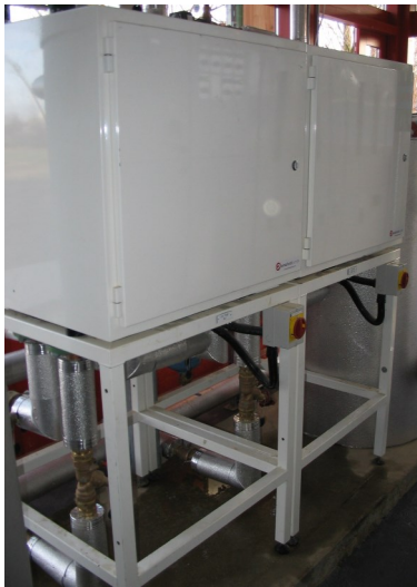
Fig 6 Plant room heat pumps
