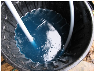
Fig 32 Slinky Purged of Air
