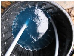
Fig 27 Slinkies Purged of Air
