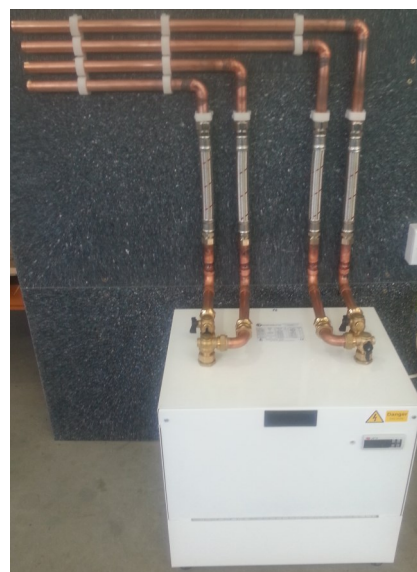
Fig 13 Shoebox with flexi connections
