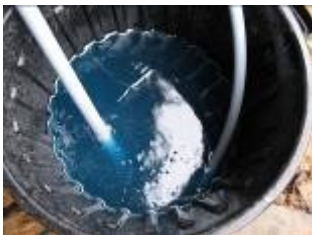
Fig 30 Slinky Purged of Air
