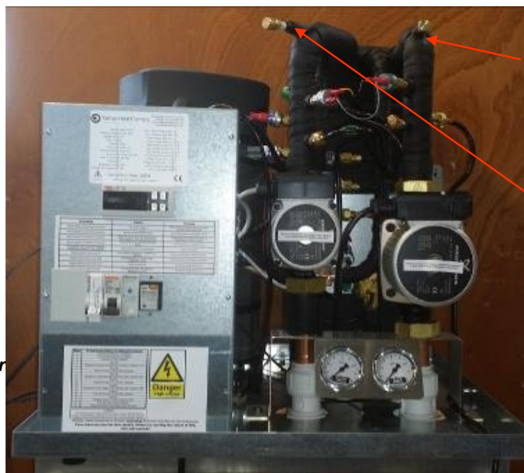
Fig 31 Location of Heat Pump Schrader Valves
