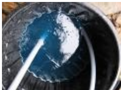
Fig 25 Slinkies Purged of Air
