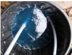
Fig 25 Slinkies Purged of Air
