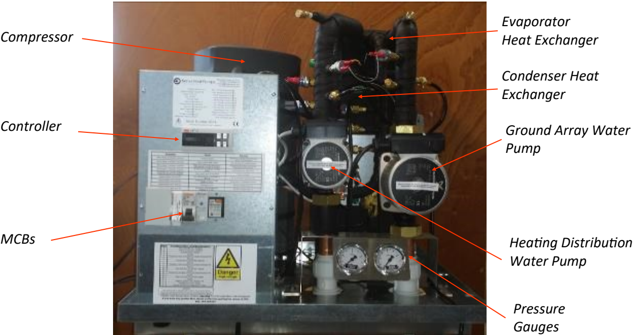
Fig 1. The internals of a heat pump
