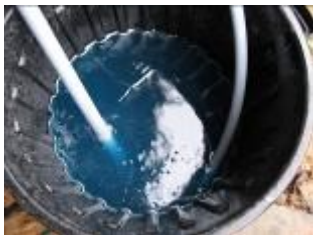
Fig 30 Slinky Purged of Air
