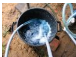
Fig 27 Purging the Slinkies of Air
