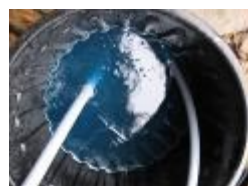
Fig 28 Slinkies Purged of Air
