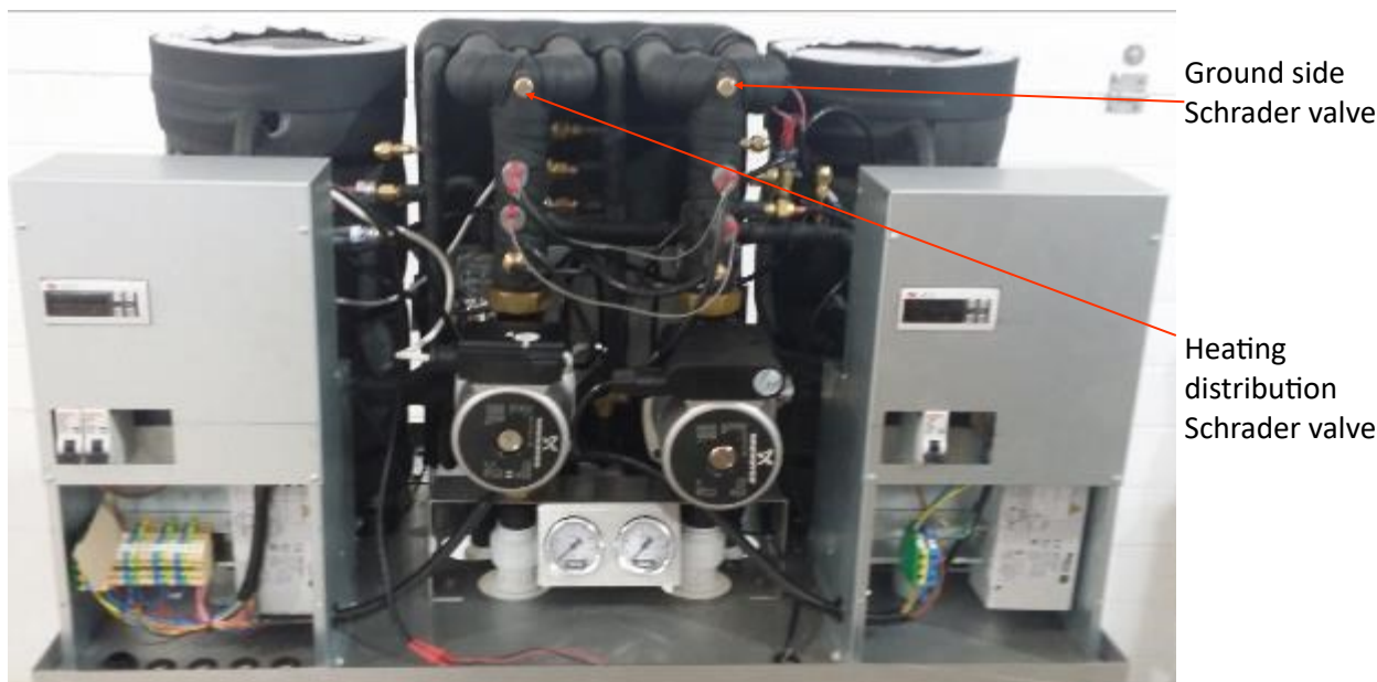
Fig 31 Location of Heat Pump Schrader Valves
