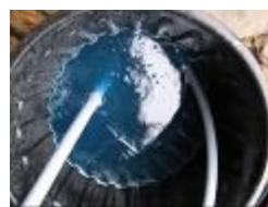
Fig 29 Slinkies Purged of Air
