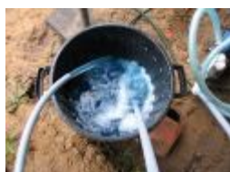
Fig 28 Purging the Slinkies of Air
