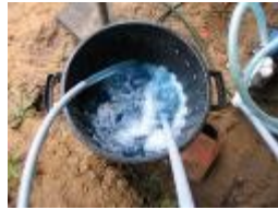
Fig 28 Purging the Slinkies of Air
