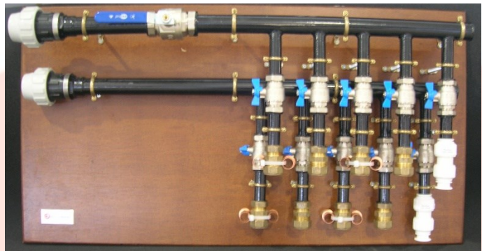
Fig 3- 4 way 'left' handed manifold
