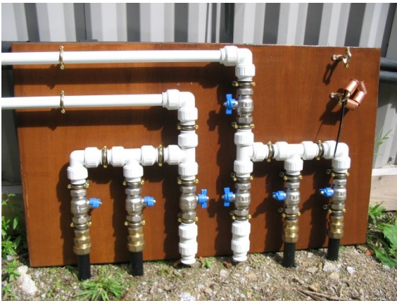
Fig 2- 2 way universal manifold (set for left handed)
