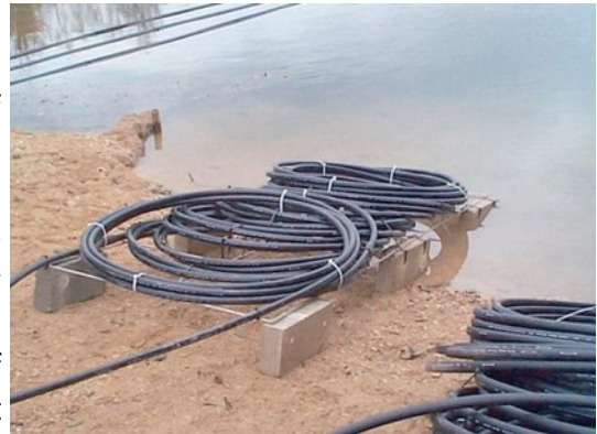
Figure 1 Installation of Pond Mats
