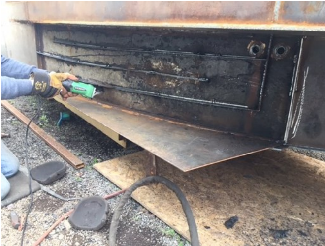
Figure 4—Skin Tank being Installed
