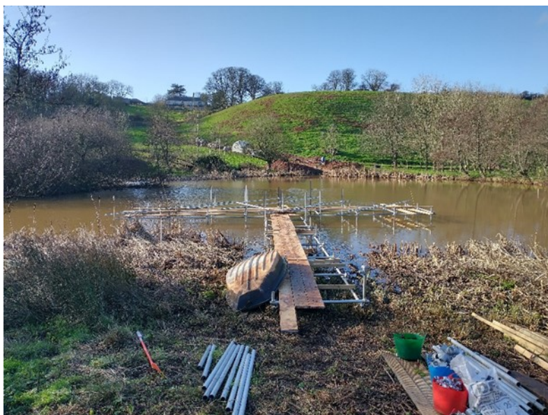
Fig 4 Bespoke Pontoon Construction
