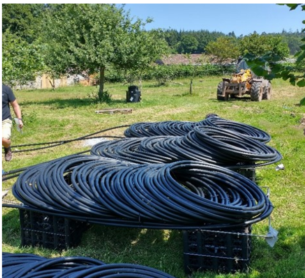
Fig 2 A pond mat with drainage crates for soft bed clearance
