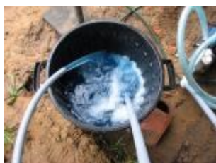
Fig 41 Purging the Slinky of Air
