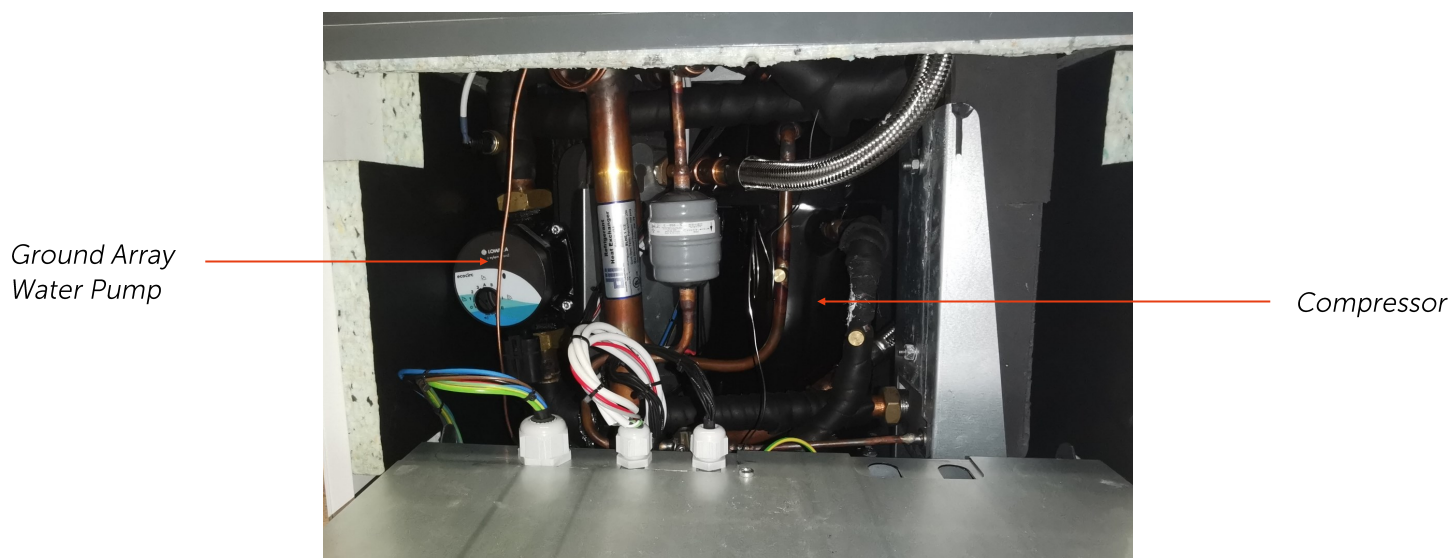
Fig 1. The internals Shoebox NX heat pump
