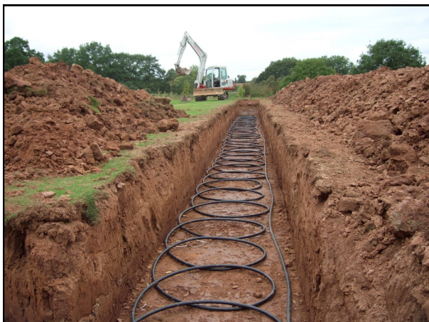
Fig 8 1.2 x 1.2m slinky installation
