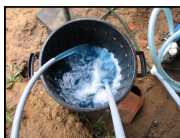
Fig 25 Purging the Slinky of Air
