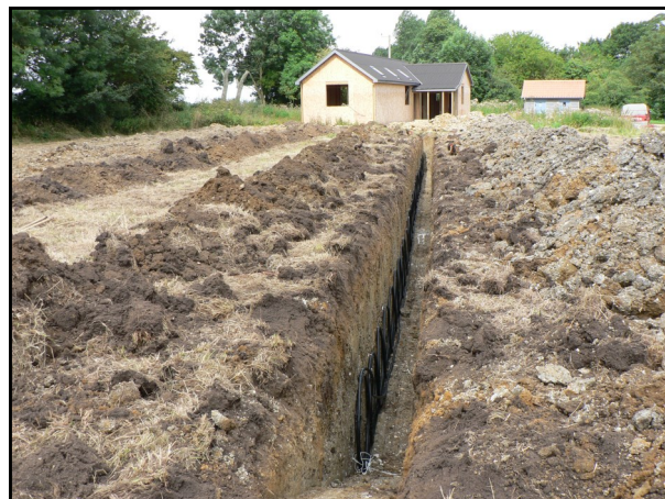
Fig 9 2m deep slinky installation
