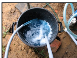
Fig 22 Purging the Slinkies of Air
