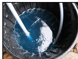
Fig 26 Slinky Purged of Air
