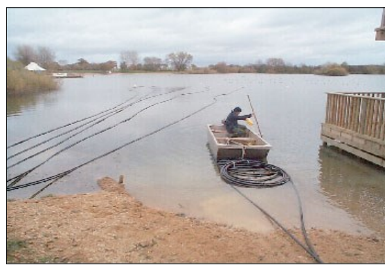
Fig 16 Floating the pond mats out
