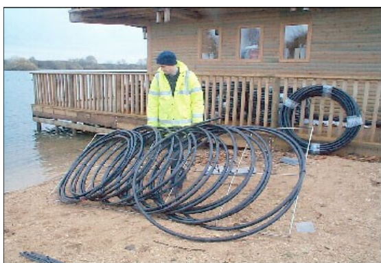
Fig 15 Slinkies mounted on a pond mat
